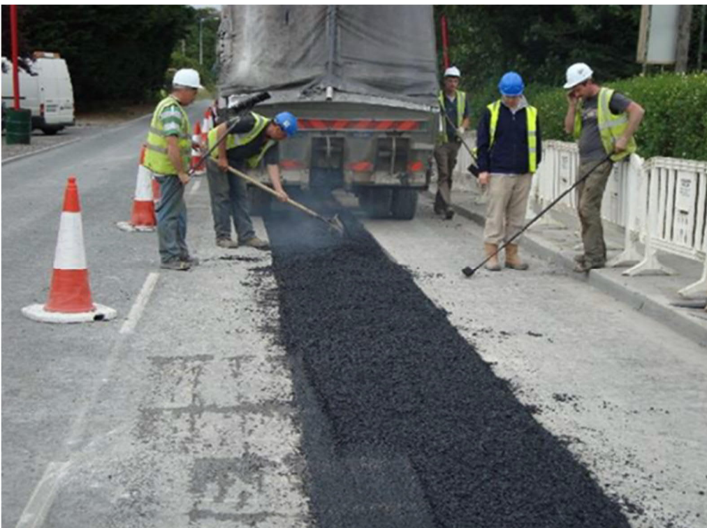
Figure 2.5: Reinstatement of Road Surface Over Trench
