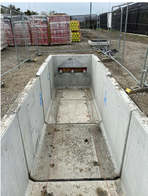
Figure 2.6: Completed Joint Bay prior to Cable Installation (pre-cast)
