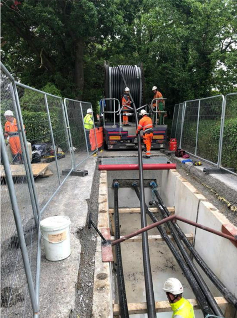
Figure 2.7: Typical Set-Up of HV Cable Pulling Procedure
